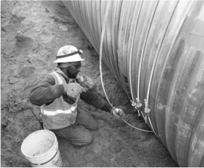
Tighten the bolts against the take up lug until the rods are tight around the pipe.
