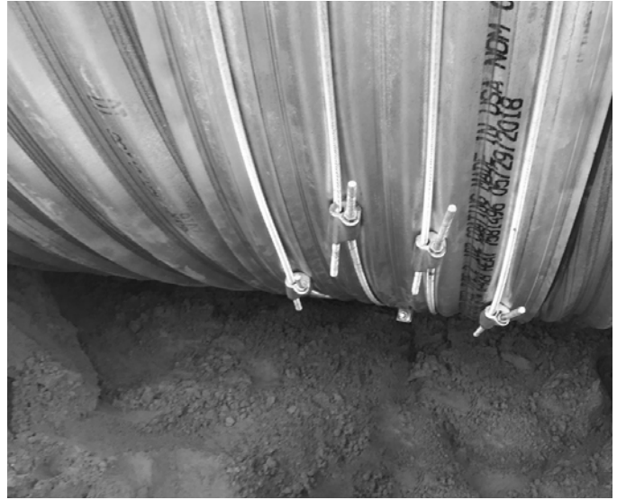
Finished levee band installation shown above.
