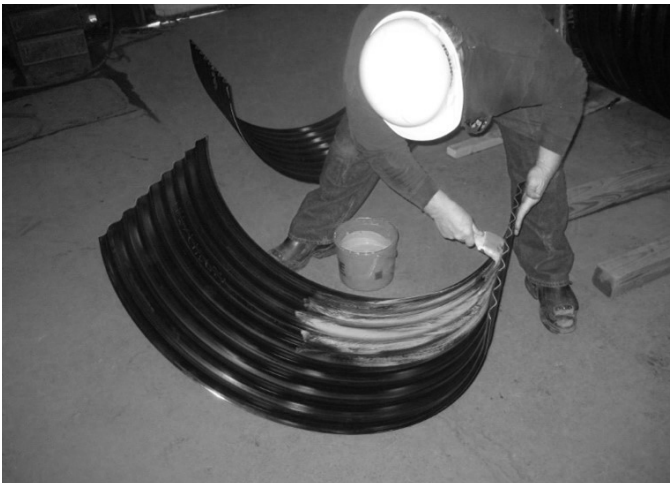
Spreading lubricant on the pipe and bands, is recommended in the area of the flat gasket for a leak resistant joint.
