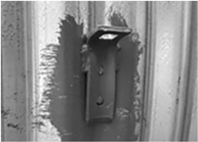
Spreading lubricant on the pipe and bands, is recommended in the area of the flat gasket for a lead resistant joint.
