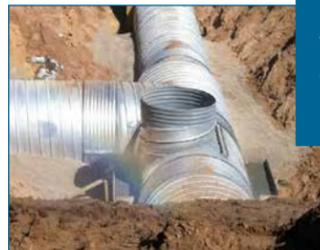
ULTRA FLO® fittings improve installation time in the field. This fitting incorporates an elbow, a riser and lateral stub. The fitting is reinforced according to NCSPA guidelines.
