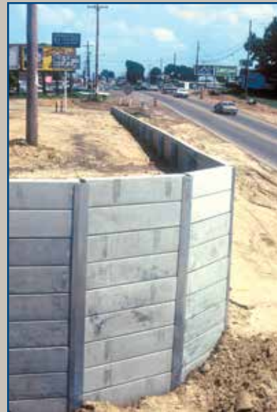
Bin-Wall system allows angle changes.
