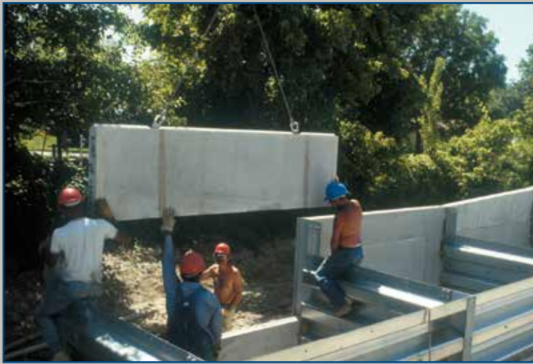
Concrete panels easily slide into place.
