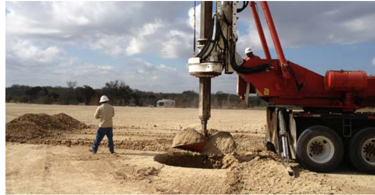
Setting the cellar occurs prior to any drilling.
