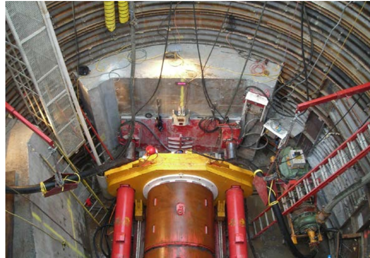
Tunnel Liner Plate Vertical Access Shafts
