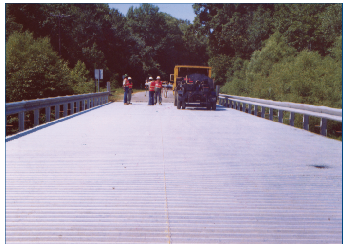
A continuous bridge deck
