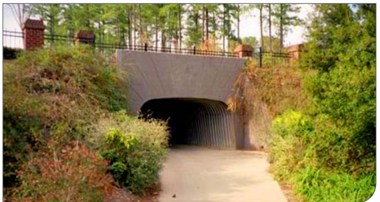
Pedestrian tunnel (OH) – allows pedestrian passage under busy roadway (ALBC)
