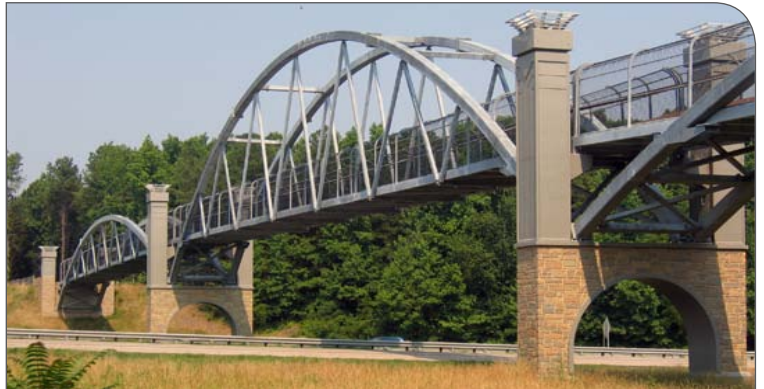
Multiple-span overpass (NC) – connects greenway system and provides safe pedestrian passage over interstate (Continental)
