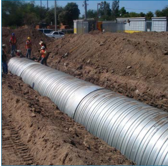
Reduced excavation because of the smaller outside diameter of ULTRA FLO®.
