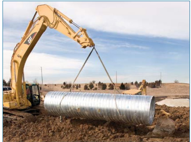
ULTRA FLO® is available in long lengths, while its light weight allows it to be unloaded and handled with small equipment.
