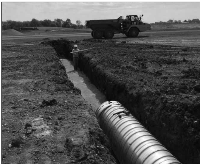
Typical storm sewer with 4" – 6" of import granular material as pipe bedding.
