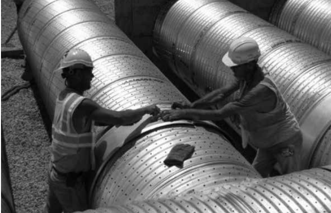
Installing a HUGGER® band on a perforated CMP
