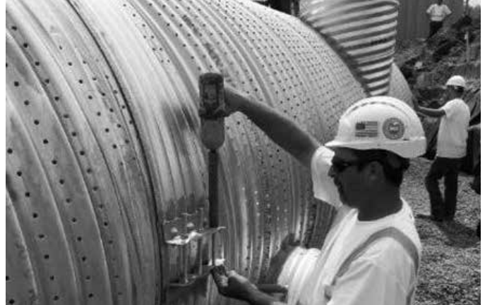
Tightening bolts on a corrugated band.
