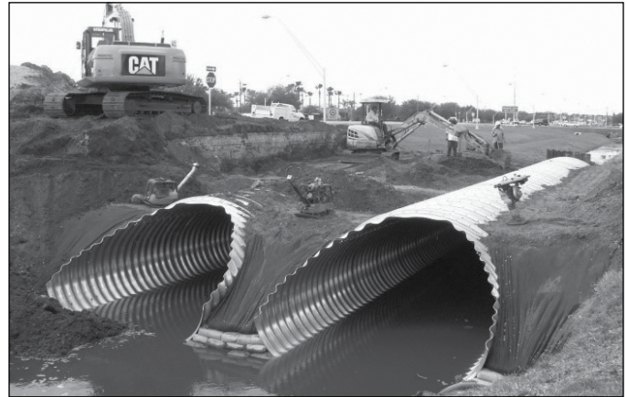
Example of backfilling for a larger pipe-arch installation.
