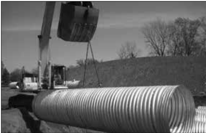
Lifting CMP utilizing factory attached lifting lugs
