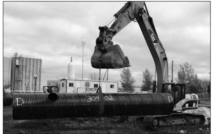
Lifting polymer-coated CMP with nylon straps
