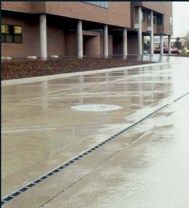
Example of an overland sheet flow.
