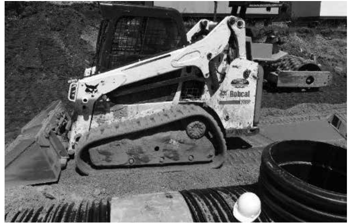
Examples of light, tracked, construction equipment used to place final cover over the pipe system.
