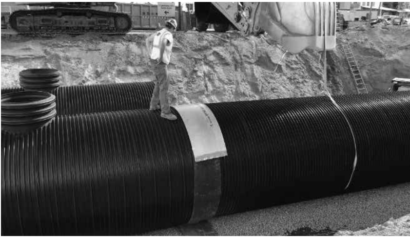
Installing a flat gasket and band around DuroMaxx plain end pipe.
