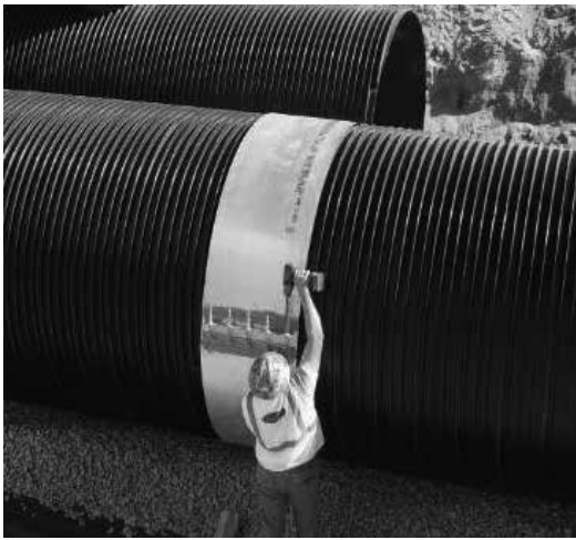
Tightening bolts on a flat band.
