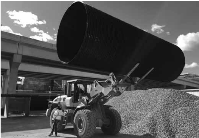
Lifting DuroMaxx off the flatbed with a frontend loader with forks.
