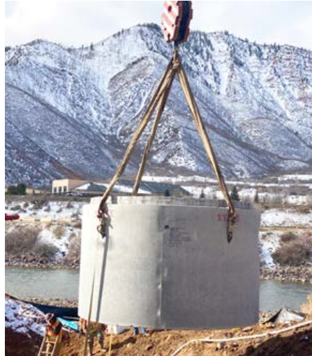
Step 2: Lift and place middle riser.
