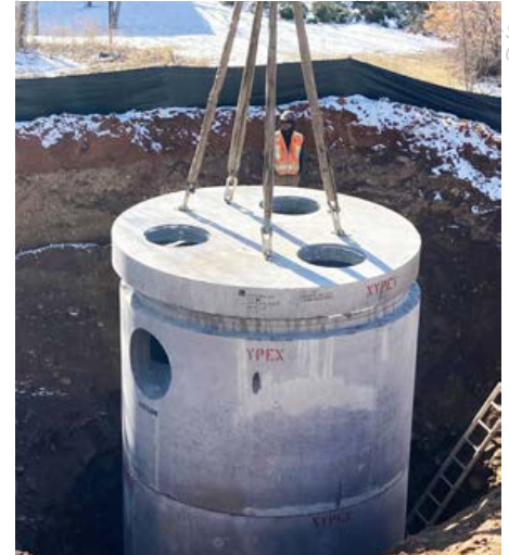
Step 3: Place top slab with access holes.
