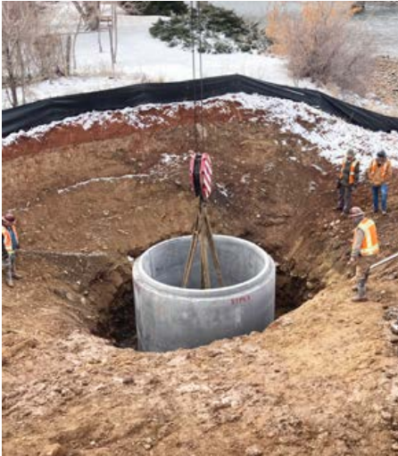
Step 1: Install the base section.
