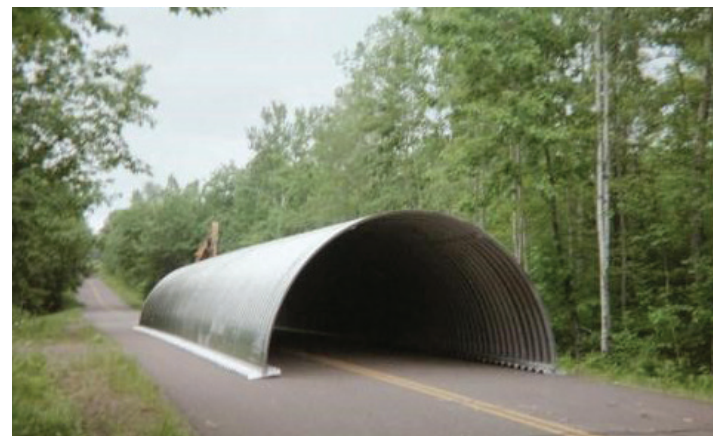
Aluminum arch on footing pads.
