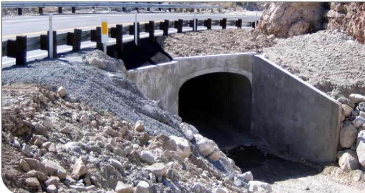
SR 18 (CA) – Caltrans emergency culvert replacement beneath popular state route (CON/SPAN)
