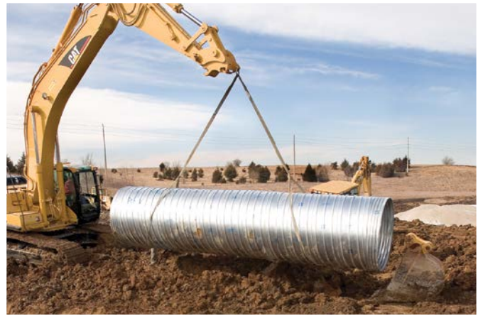
ULTRA FLO®, a pipe with a smooth interior, is the material of choice for storm sewer applications and a lower cost alternative to reinforced concrete pipe.
