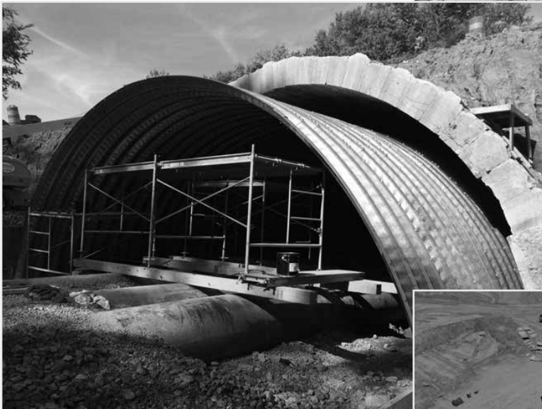
BridgeCor Reline of Old Stone Arch Bridge
