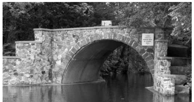
72-Year-Old Steel Structural Plate Pipe Arch Installed c. 1940 | Inspected in 2012
