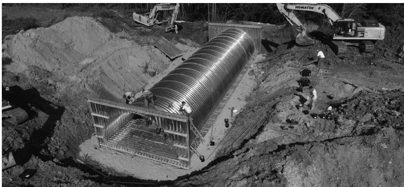
Assembly of Aluminum Structural Plate with Headwalls
