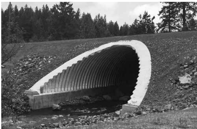
BridgeCor Arch with Full-Beveled Ends and Slope Collar
