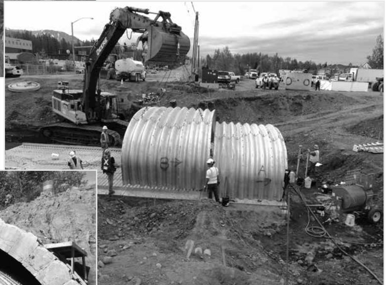
BridgeCor Box Culvert Assembly
