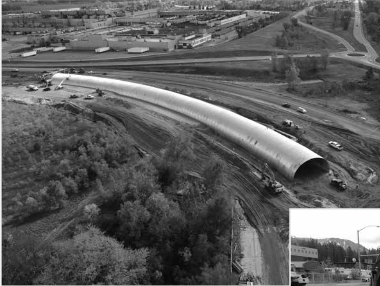
BridgeCor Tunnel Installation
