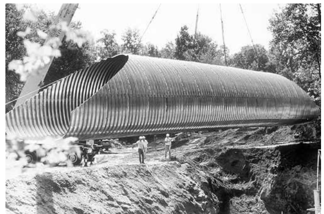
Lifting of Assembled Aluminum Pipe Arch
