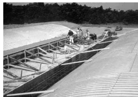
Horizontal reinforcement bars are tied to Contech bent and threaded rods to provide reinforcement for the concrete thrust beam.
