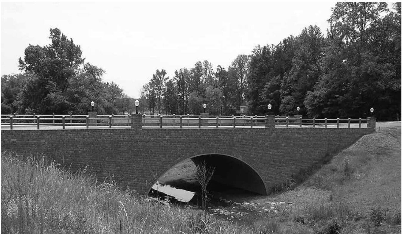
SUPER-SPAN Single Radius Arch with Keystone Headwalls for a Residential Development.
