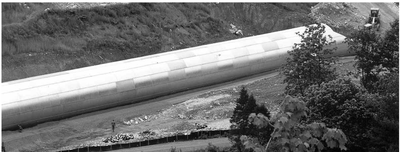
24'-0" diameter steel MULTI-PLATE® designed for 60 feet of fill owned by VDOT in Dryden, Virginia
