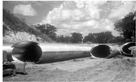
Installation of Aluminum Horizontal Ellipses
