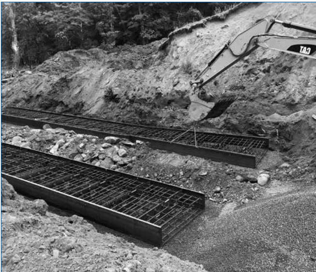
Set footers in place
