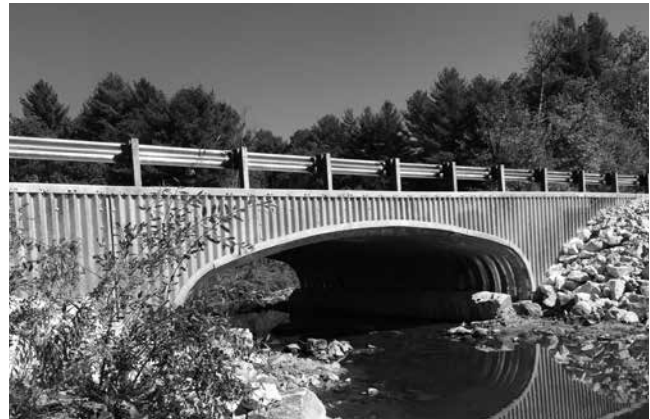
BridgeCor with Bolt-A-Plate® Metal Wall End Treatments
