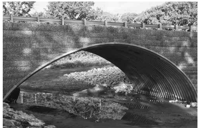
BridgeCor with Welded Wire Wall System
