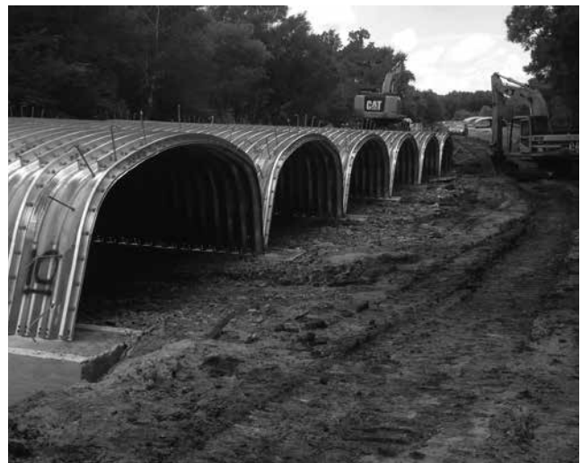
Aluminum Box Culvert multi-cell installation
