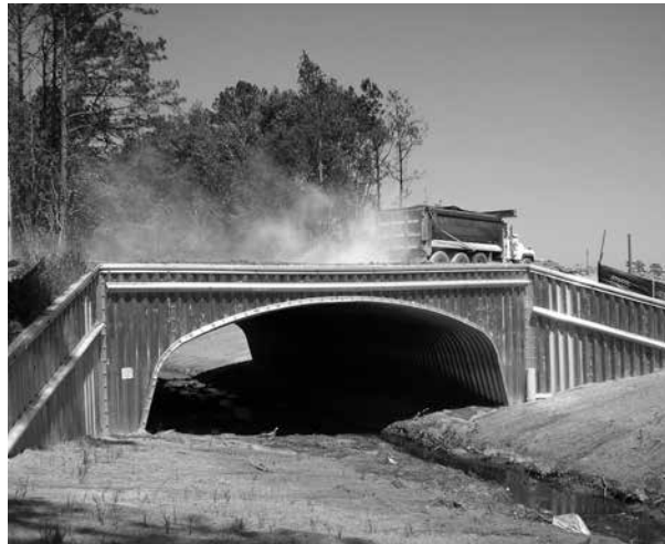
Aluminum Box Culvert with Full Aluminum Headwall Package
