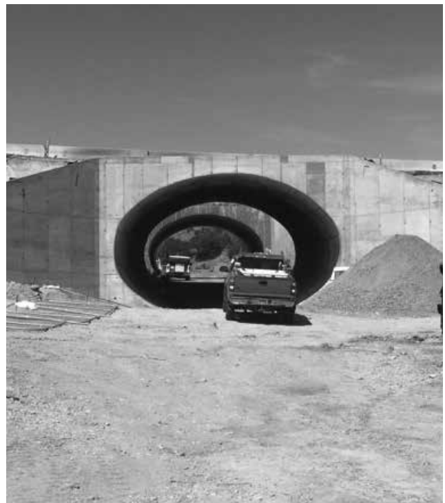
SUPER-SPAN horizontal ellipse with reinforced concrete headwall for a mining application.
