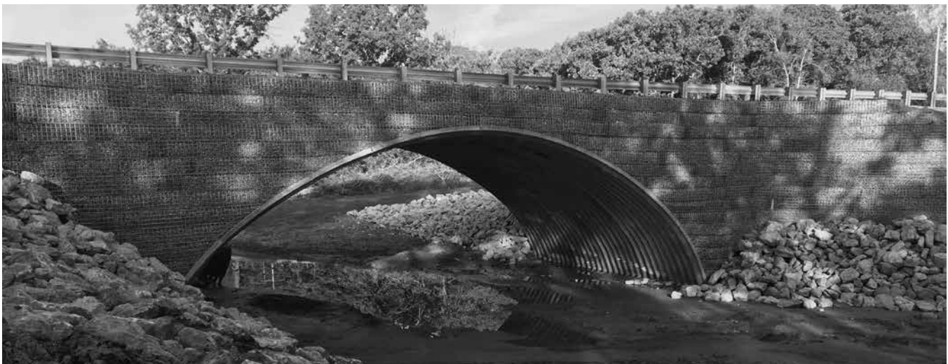
BridgeCor with a welded wire wall system for a county road stream crossing.
