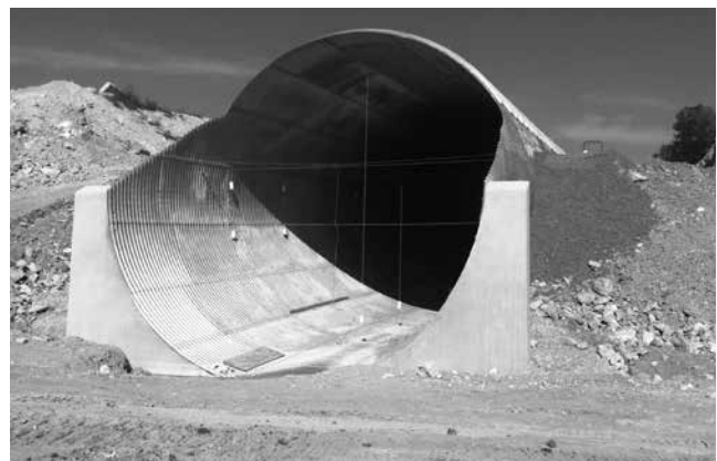
MULTI-PLATE® with Step-Beveled End and Concrete Collar
