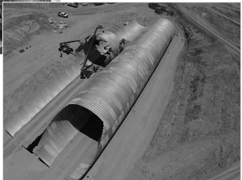
BridgeCor Assembly
