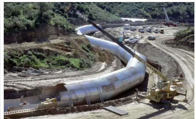
Structural Plate installed along curved alignment.
