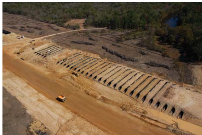
Polymer coated HEL-COR® is used to withstand corrosive soil conditions.
