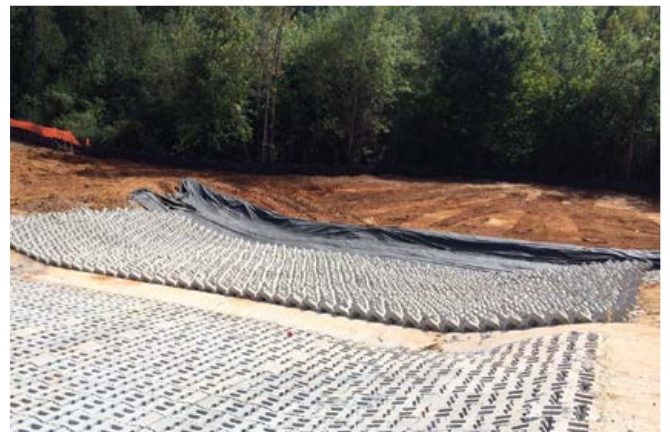
A-Jacks rapidly dissipate energy before flow transitions to natural environments.
