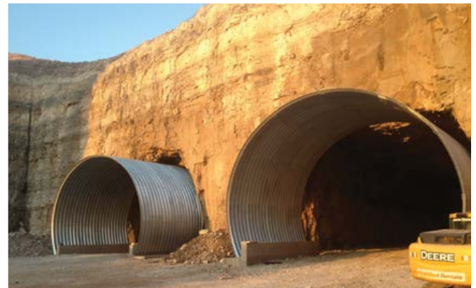
The strength-to-weight ratio of BridgeCor® makes it a cost-effective and structurally efficient solution for limited access roads.
