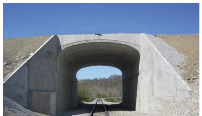
Combination of precast concrete arch elements, headwalls and wingwalls.
