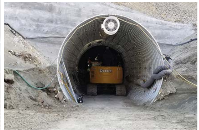
2-Flange Liner Plate offers superior plate stiffness and seam strength and the ability to construct from inside the structure.
