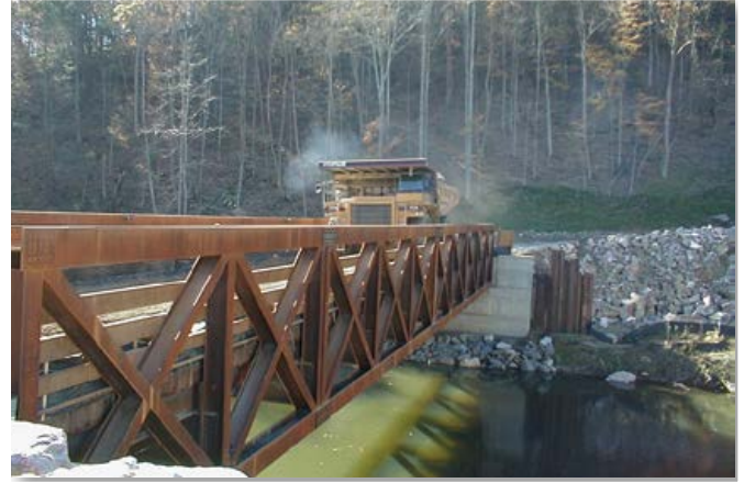
Weathering steel Steadfast vehicular truss supports heavy construction equipment in West Virginia.
